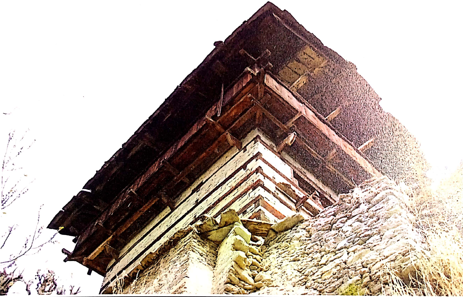
Fig. 7: Raised platform erected over in situ rocks to support the multi-storied structure.
