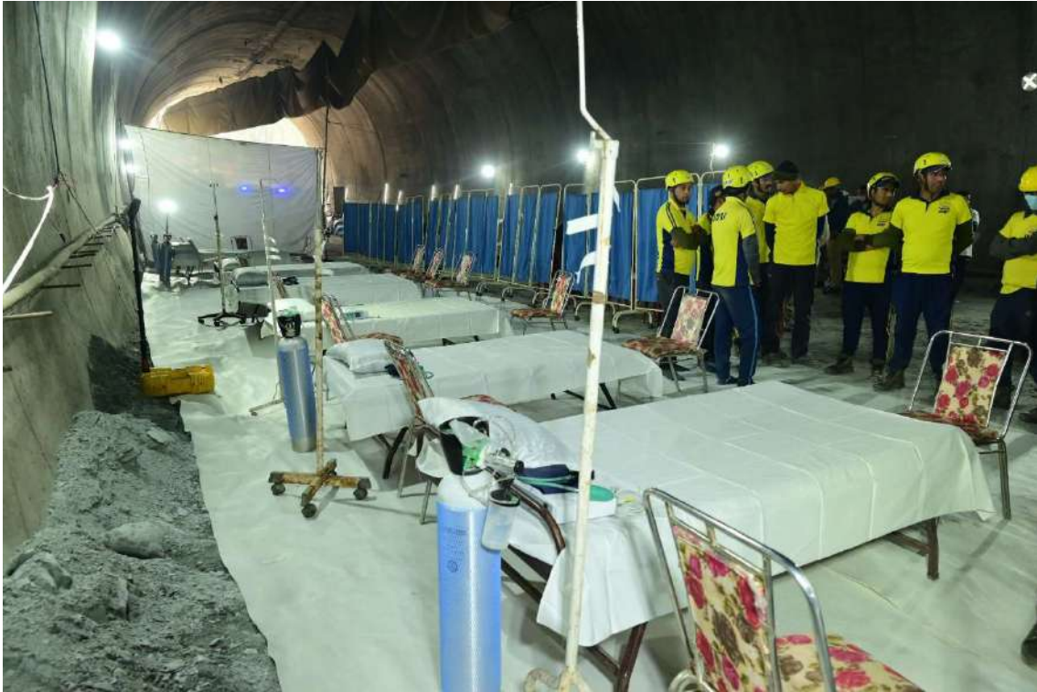
In Figure 21, The image showcases the health facilities available at the site for the well-being of those affected. the medical team is prepared, and beds have been arranged to accommodate all individuals who were trapped.
