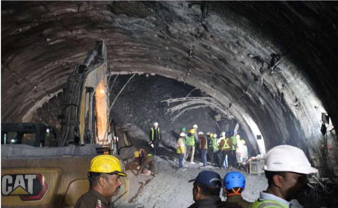
Figure 7 illustrates the conditions within the tunnel on December 14, 2023.
