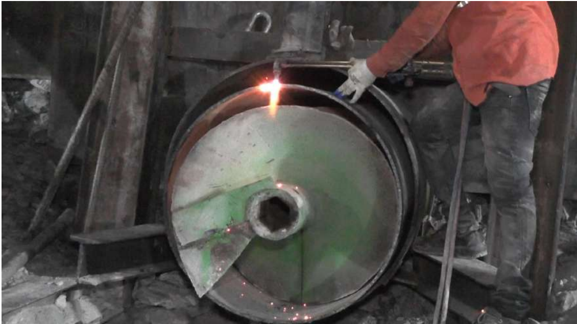
In Figure 13, the initial pipe has been connected and seamlessly inserted, marking a pivotal stage in the bindings process.
